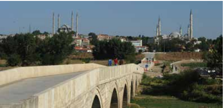
The Bayezid II Bridge over the Tunca River which connects the Bayezid II complex with the city center.
