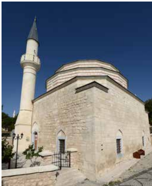
Hasan Bey Mosque, as a work of the 14th century
