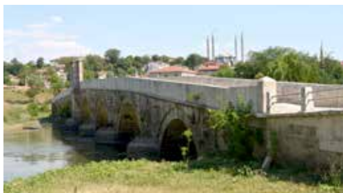
Saraçhane Bridge located over Tunca River
