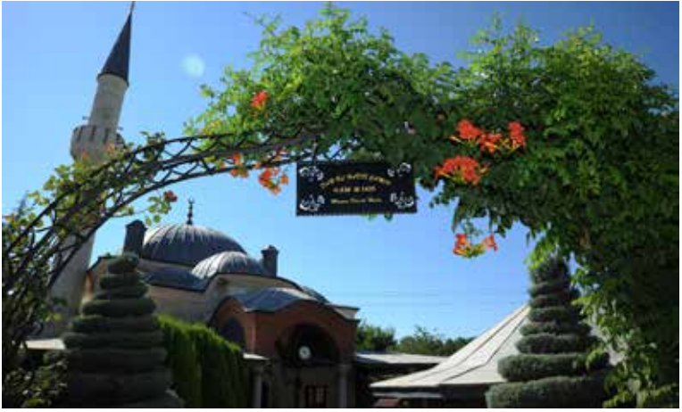
Dar'ül Hadis Mosque has carried the award of "The Most Environmental Mosque" since 2000
