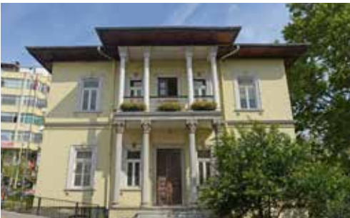
Old Municipal Building
