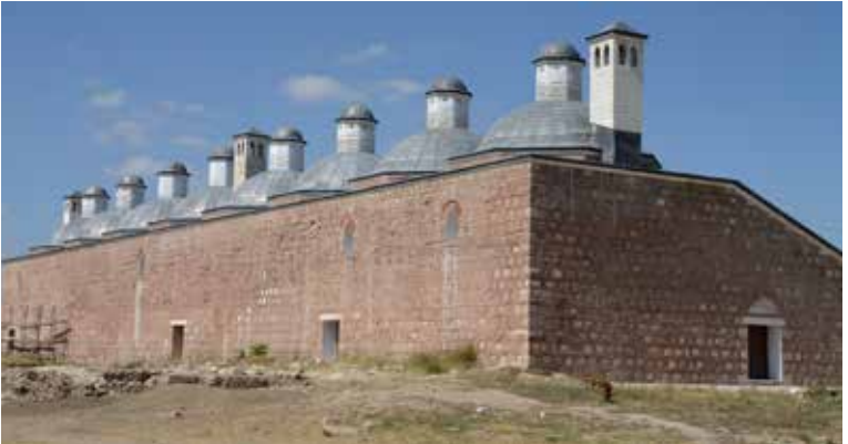
Matbah-ı Amire where palace meals were prepared was restored and regained its old look.
