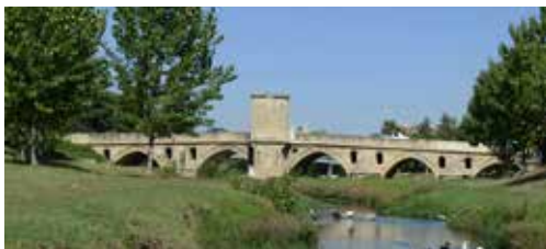
Babaeski Bridge which is located at the entrance of the town
