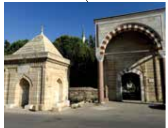
Gate of the Complex: The Gate of the complex opens to the yard of the mosque and the Sinan Ağa Fountain.
