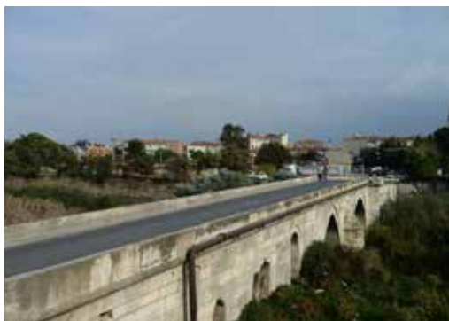
The historical Sokollu Mehmet Paşa Bridge is still used today
