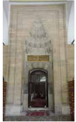
Rüstem Paşa Mosque entrance gate
